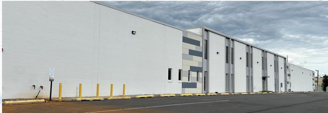
Warehouse and Offices- 200 Maltese Dr., Totowa, NJ
